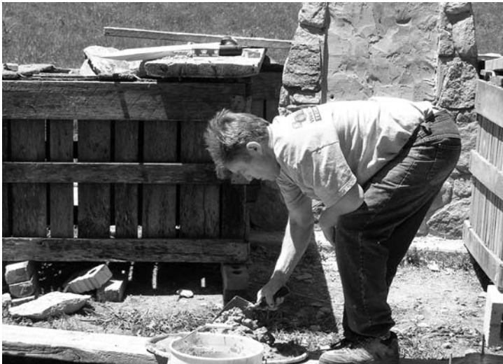
Warner Martin mixes some "mud" to cement the fieldstones into place on the mill cairn.
